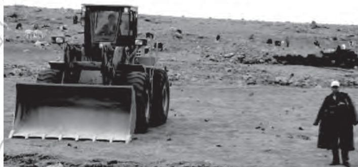
Chinese worker involved in the Ethiopian road building program
